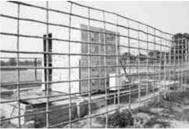
Fig 72: Maple has installed a sewage treatment plant that runs on electricity.
