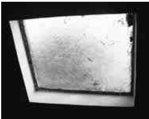
Fig 46: Jungle lodge has inserted skylights in the verandah and toilets completely eliminating need for light during the day in these spaces.
