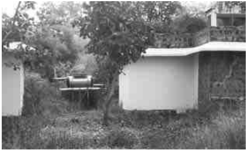
Fig 73: Camp Mewar has a series of tanks with sand gravel filters where the water passes before being let off into a water body
