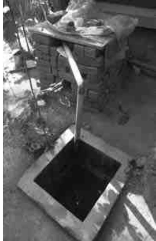
Fig 35: Jungle Lodge has created a small tank that takes the water overflow from the overhead tank. This in turn is used to water plants.
